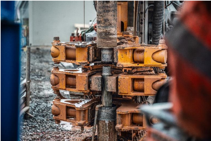
(3) Three drilling teams worked on the site.
